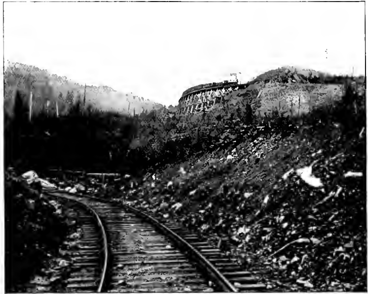
CROWN TRESTLE NEAR ROSSLAND, B. C.
